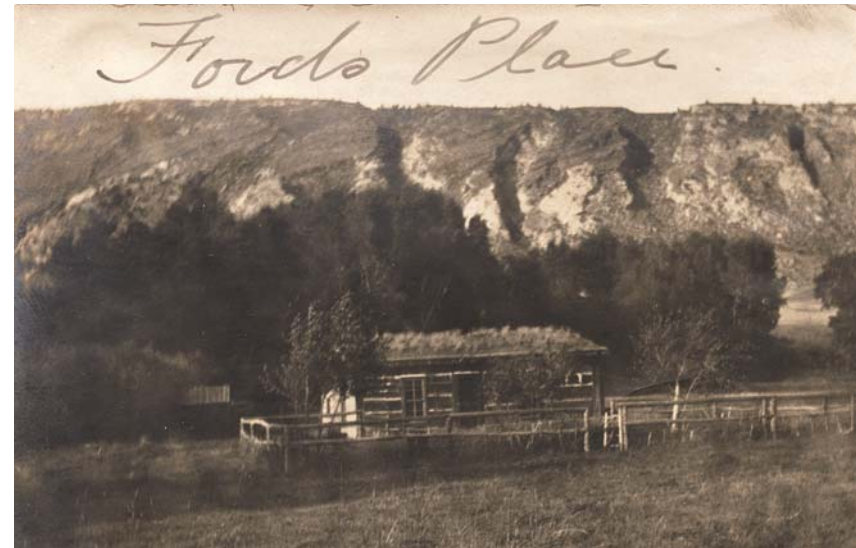
Located near Ten Sleep, this small ranch or farmhouse appears to have been a part of the homesteading wave of the 1890s and 1900s. The date of the photograph is unknown but was prior to 1909. Note the sod roof on the log house. Photograph from collection of Michael Cassity.
