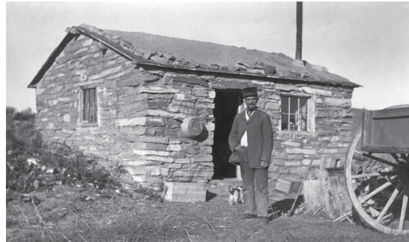
The use of locally available building materials on a small operation is evident in this USGS photograph of homesteader Jack Hooten and his cabin, in the Rock Springs USGS quadrangle. Photograph: A. R. Schultz, USGS Photographic Library, Schultz, A. R. 0527 sar00527. Although undated, the image was probably made in 1907 when Schultz made other photographs in this area.
