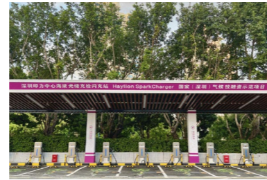
Integrated fast charging station for optical storage and charging inspection equipment
