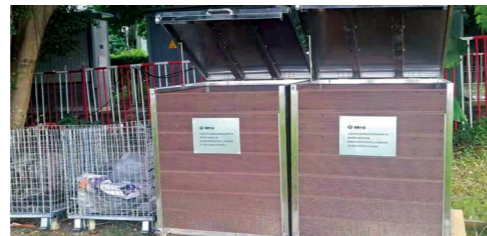
A compost station set up under the big banyan tree, including compost bins and transfer cages for temporarily storing green waste
