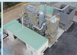
Fukushima Hirata Biomass Power Unit No. 2
