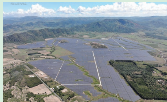
Output: 214 MW (Shikoku Electric Power's share: 32 MW)
