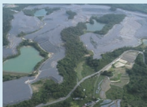
Bizen Kumonoue Solar Power Plant
