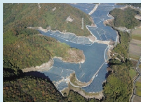
Yumesaki Yumefurusato Solar Power Plant
