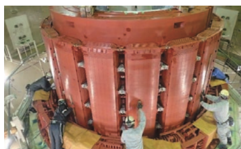
Hanging the generator rotor
