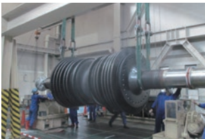
Lifting the high pressure turbine
