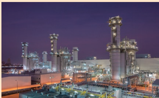
Output: 1,800 MW (Shikoku Electric Power's share: 270 MW)
