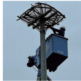
Inspection and maintenance of nesting towers (Seiyo City)
