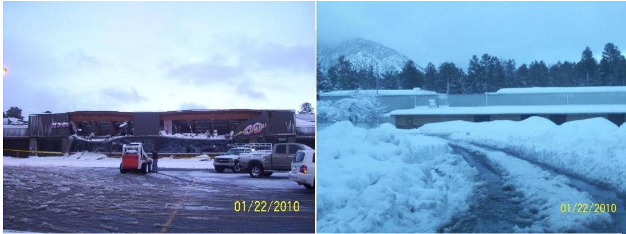
Fig. 24. Roofs of several business in Flagstaff collapsed, including a fabric and bookstore (left), and a community ice rink (right).
