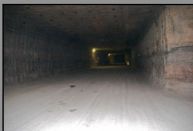
Openings are mined 2,150 feet underground in the ancient salt formation.
