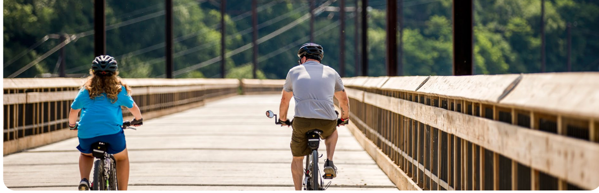
Enola Low Grade Trail Trestle Bridge in Pennsylvania.
