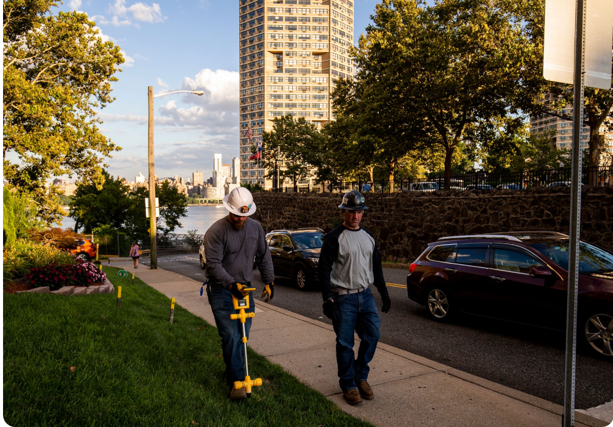
Michael Post and Michael Pyskaty, New Jersey Operations Technicians marking pipelines.
