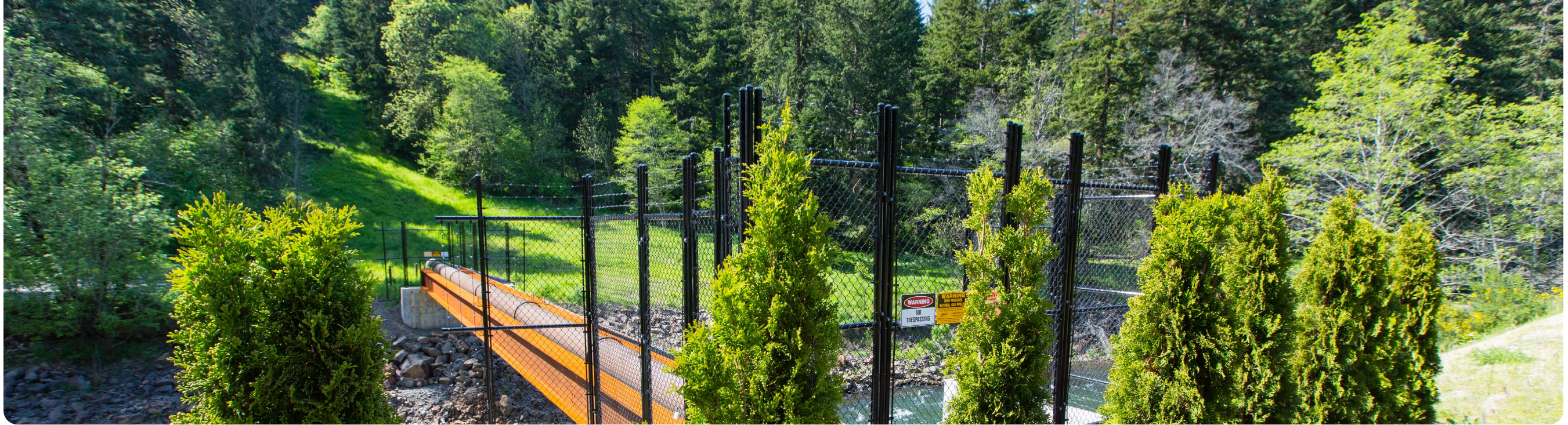
Northwest Pipeline in Hood River, Oregon.
