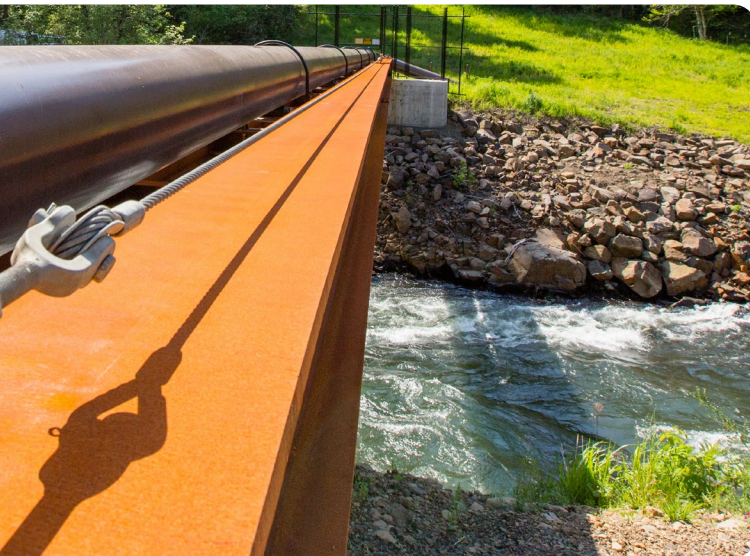
Northwest Pipeline in Hood River, Oregon.
