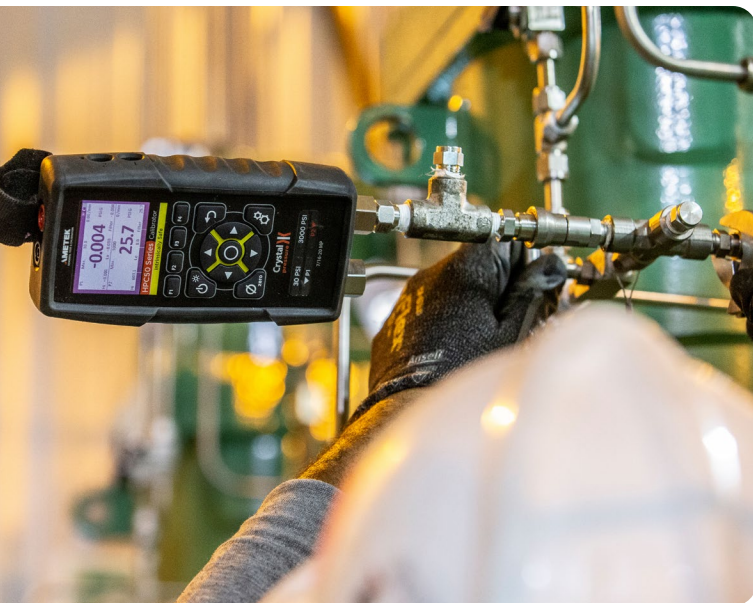
Metering station in New York City.
