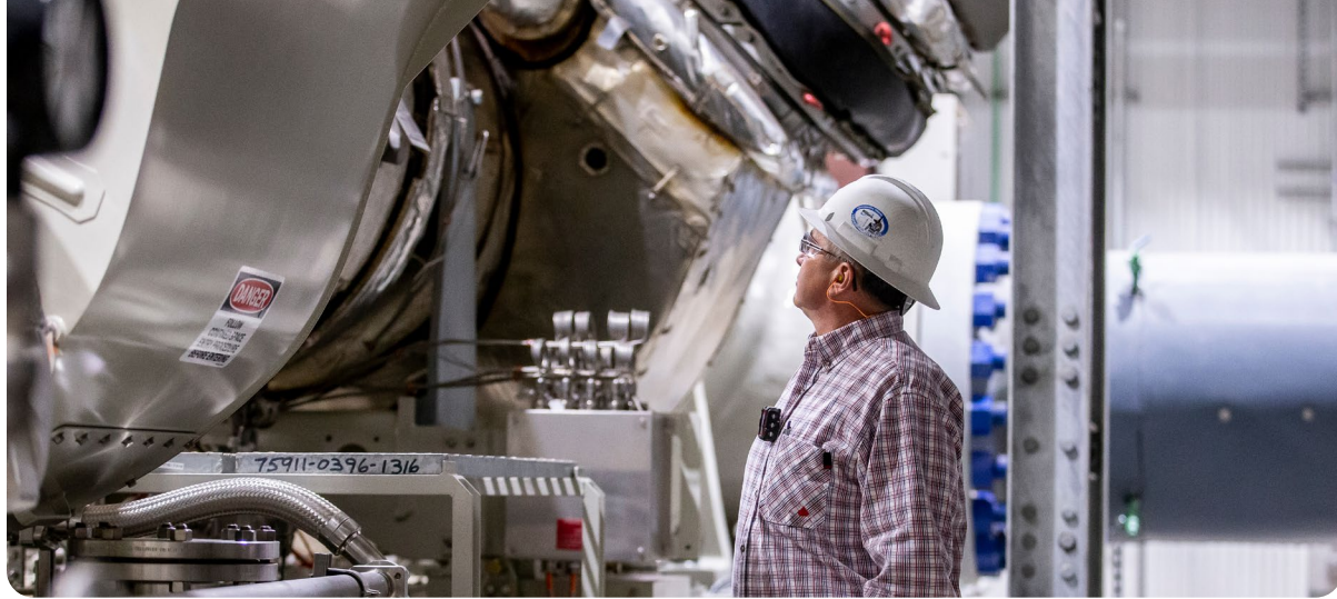
Jerry Oakes, Operations Supervisor, at Compressor Station 165 in Virginia.
