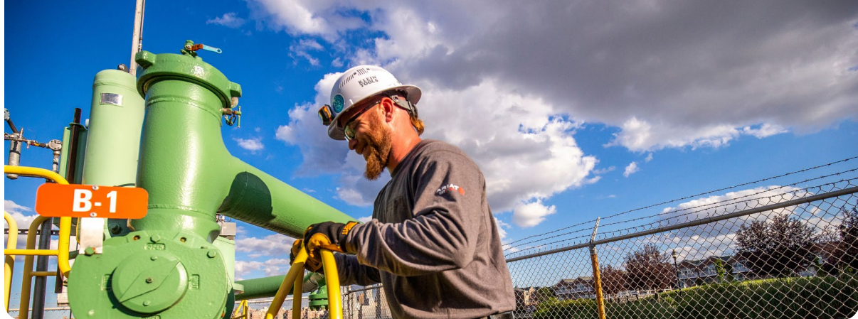
Michael Post, Operations Technician at 72nd Street Metering Station in North Bergen, New Jersey.
