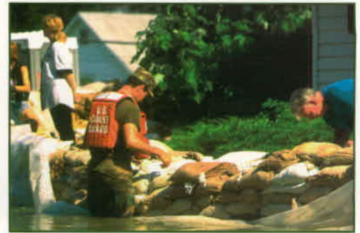
▲ Photo: Federal Emergency Management Agency
