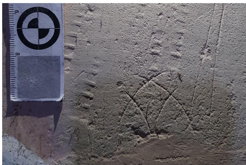
Figure 16: Architectural design for window tracery from St Michael's, Betchworth. (Photograph: Author)
