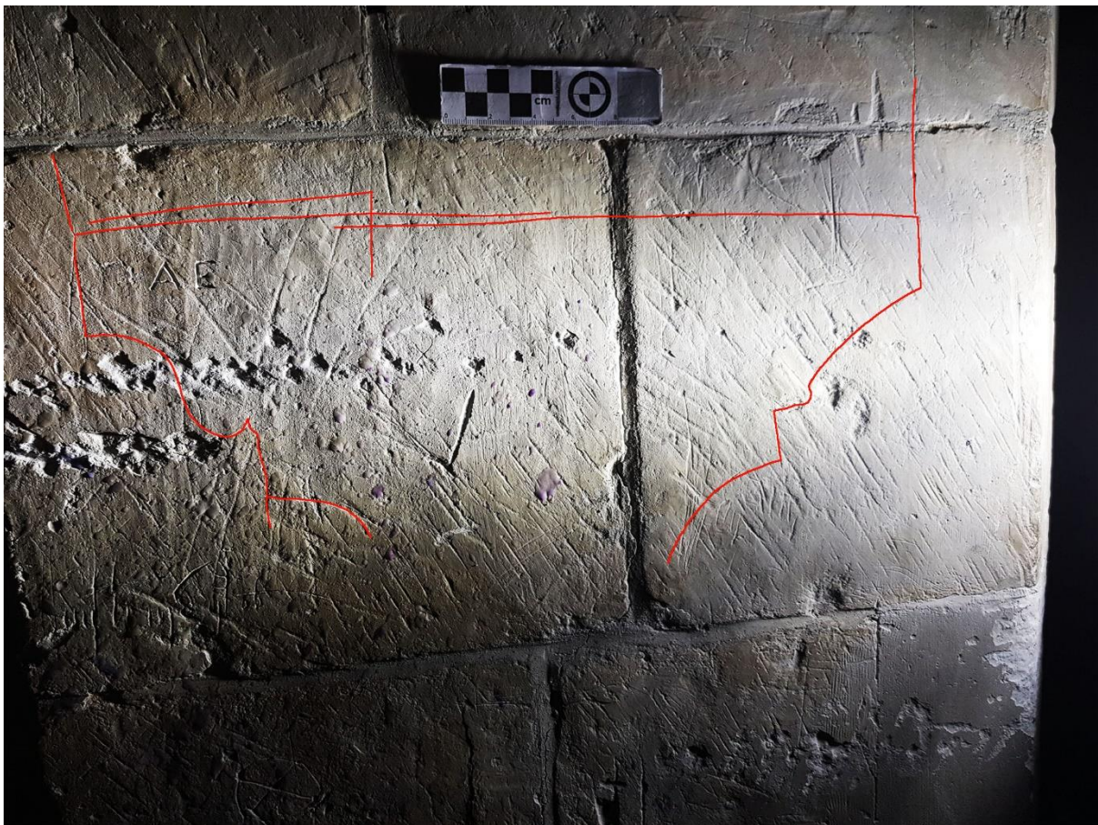
Figure 18: Architectural designs of window jamb mouldings in profile from St Nicholas, Pyrford. (Photograph: Author)
