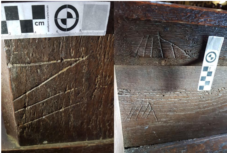
Figure 15: Examples of carpenter's marks found on 13 th century pews at St Mary and All Saints, Dunsfold. (Photographs: Author)
