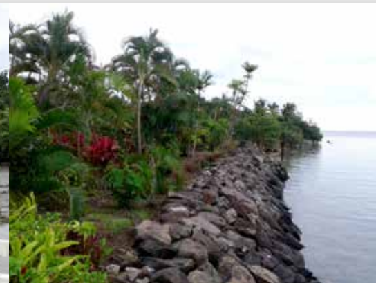
Removal of mangroves impacts on fish stocks and coastal stability, installation of stone seawalls for coastal protection needs to be carefully planned and assessed through a robust EIA prior to implementation, to ensure they will effectively protect community assets and not cause unintended impacts along neighbouring areas of coastline. Photo: Greg Barbara
