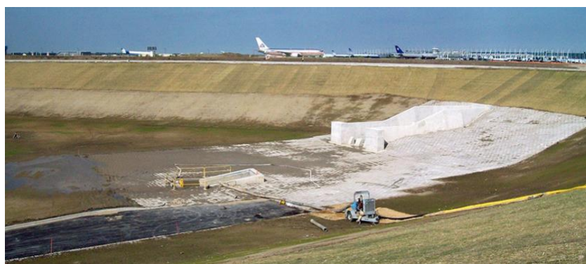
Figure 7: Expansion Works on Flood Retention Basin at Chicago O'Hare Airport 235
