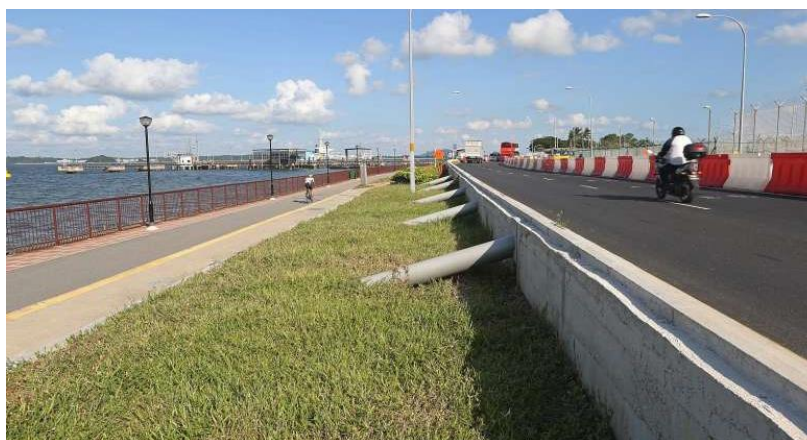
Figure 6: Road Doubling as Seawall at Singapore Changi Airport 226
