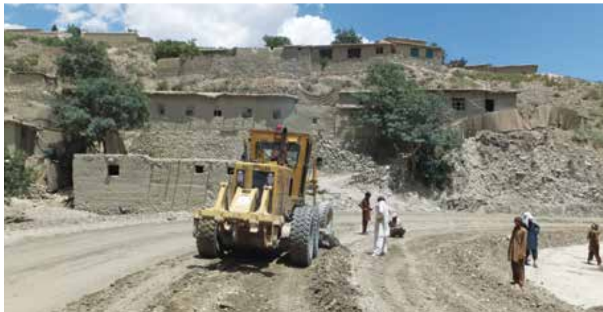
Workers grade an Afghan roadbed for a USAID-funded project. (USAID photo)
