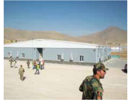
The new IT building , part of the second phase of Marshal Fahim National Defense University in Kabul. (U.S. Army Corps of Engineers photo)
