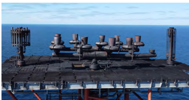
From left to right Bruce platform HP Flare tip, manifold and LP Flare tip
