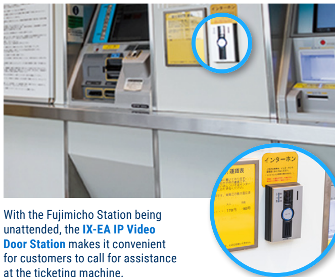
At the Ofuna Station ticket office, the IX-MV7-HB IP Video Master Station makes it possible to respond to customers at unattended stations while having the option to view video from the door station or the network camera.
