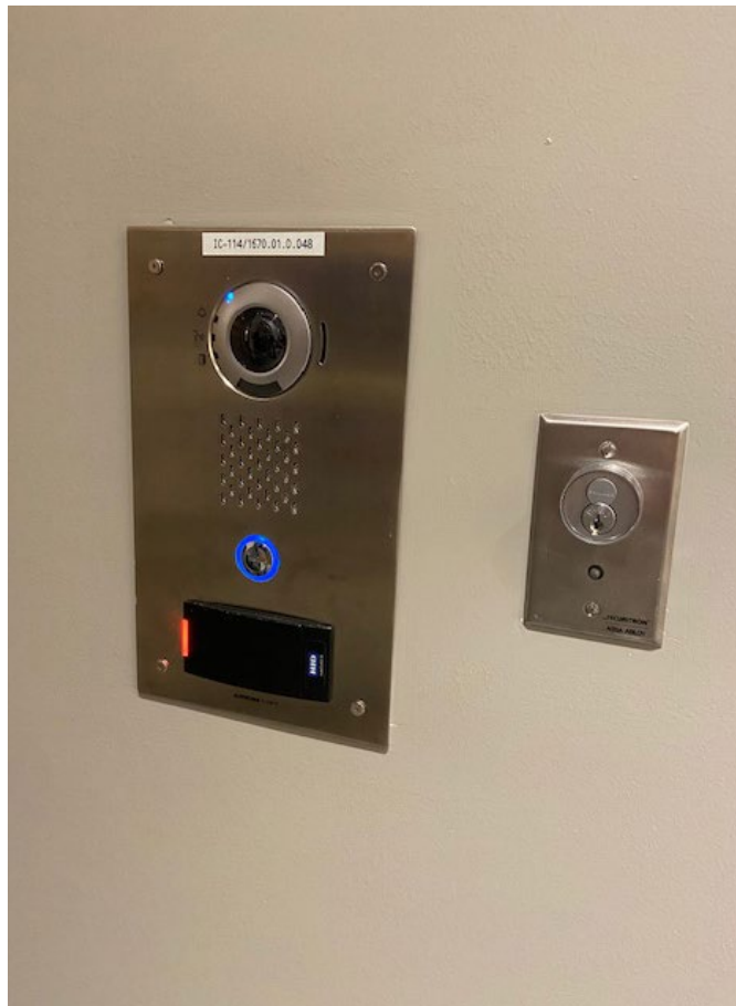
For convenience and security, the Card Access IP Video Door Station (IX-DVF-P) , allows staff with badges to access authorized-only locations.
