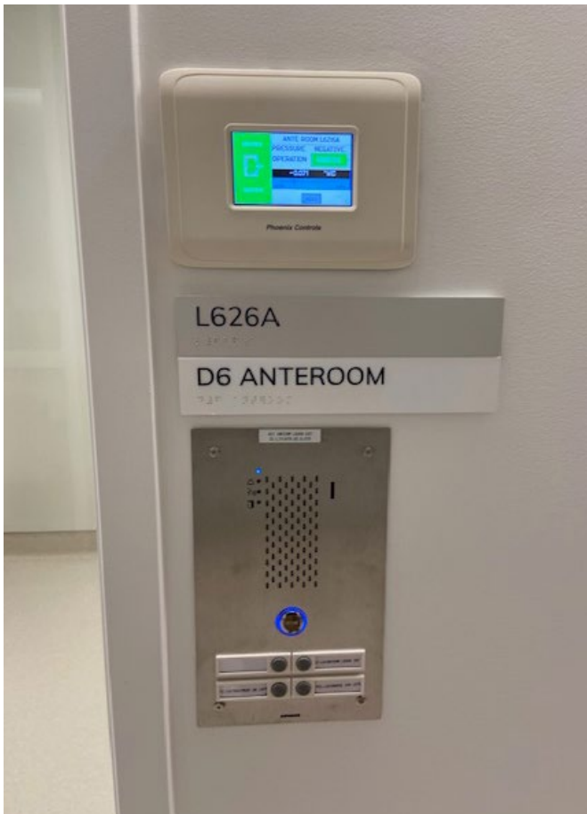
To meet the needs of Oak Pavilion, Aiphone's unique 4-Call IP Video Door Station (IX-DVF-4) was specially customized for their anterooms.
