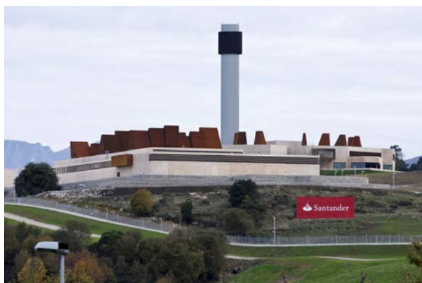
Data centre Cantabria
