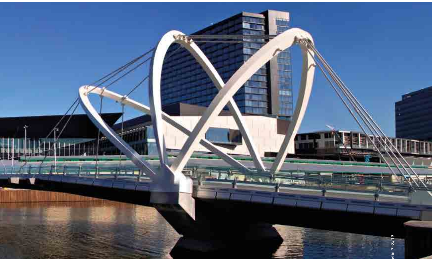
Modern footbridge over the Yarra River at Melbourne's Convention and Exhibition Centre.
