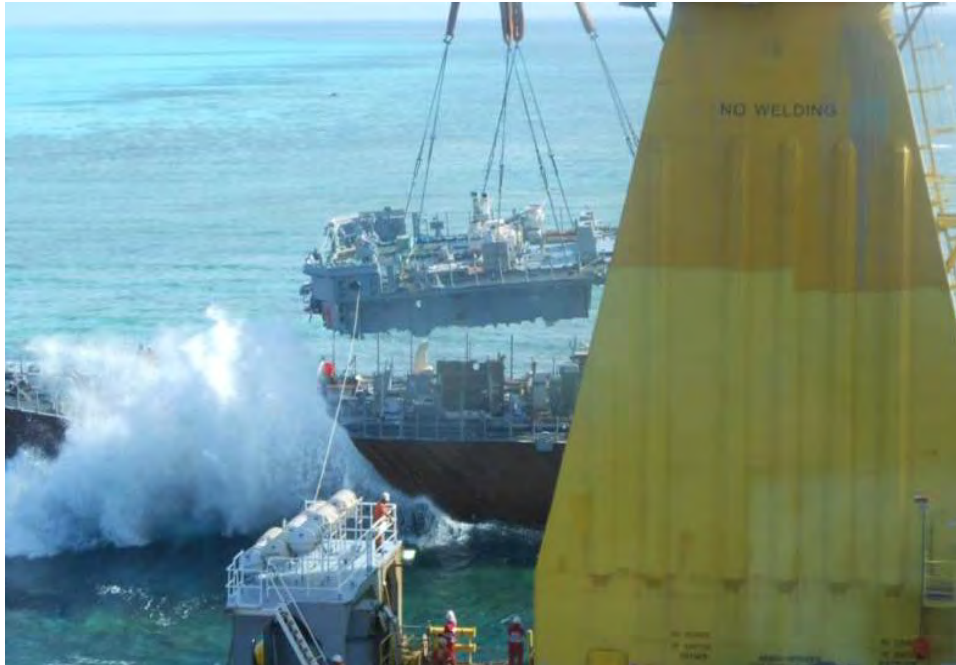
Figure 5-14. 01 level forward being lifted off GUARDIAN. Note waves breaking on hull. This lift followed a number of days where high waves prevented operations on GUARDIAN.
