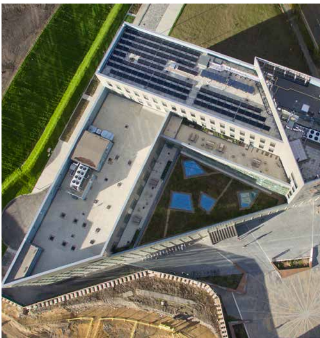
Newcastle Urban Sciences Building
