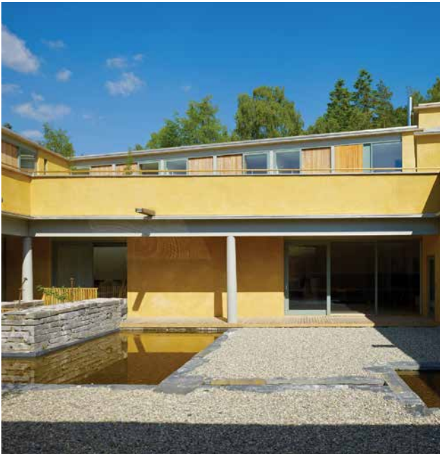
WISE Building External view
