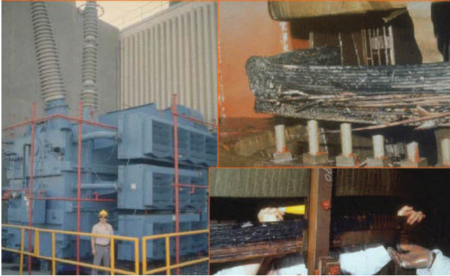
March 1989 magnetic storm damage to a high-voltage transformer at a nuclear power center in Salem, New Jersey.
