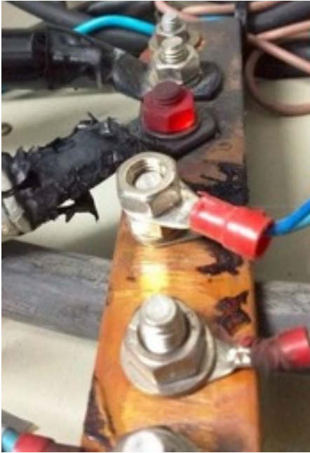
Loose connection leads to overheating / glowing connection
