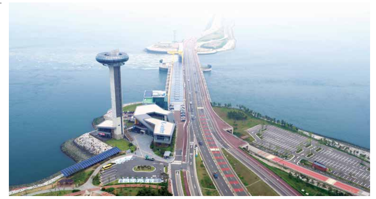
Sihwa Lake Tidal Power Plant
