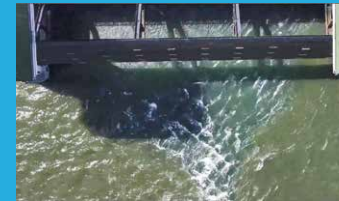
Seawater inflow (undercurrent)
