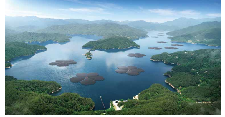
Hapcheon Dam Floating Solar Power
