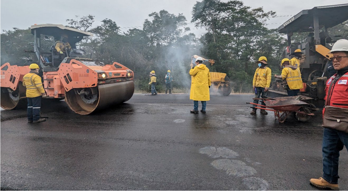
Photo 4. PPE used by contractor workers
