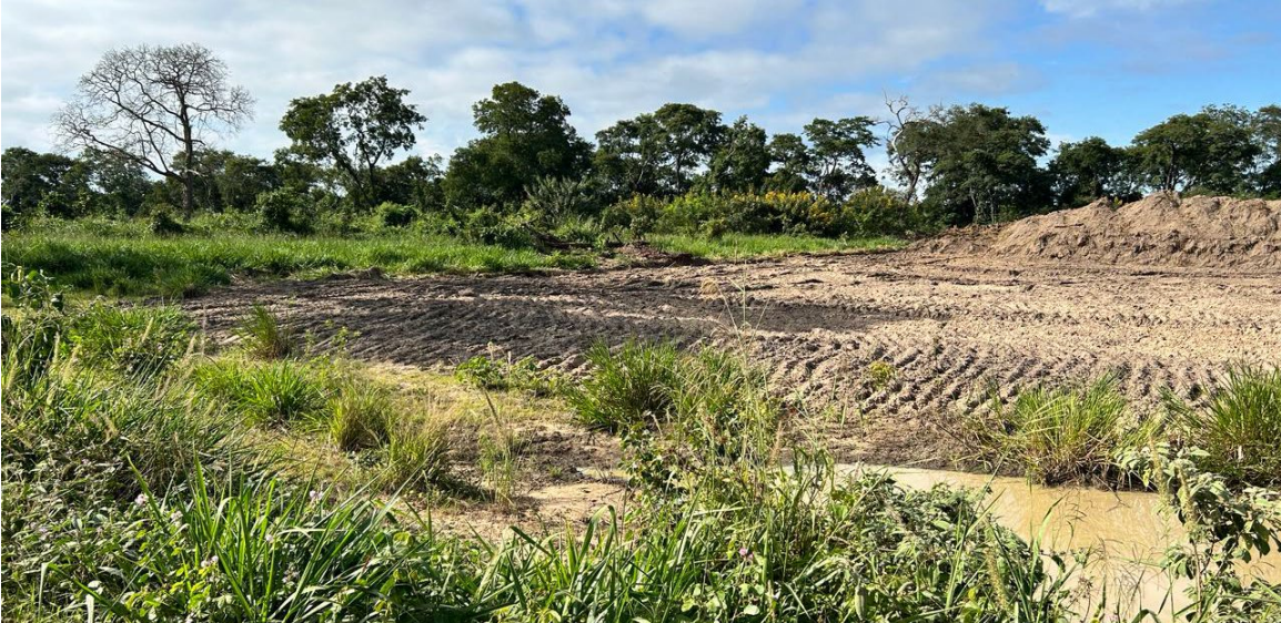
Photo 1. Borrow pit site in process of closure, pending revegetation
