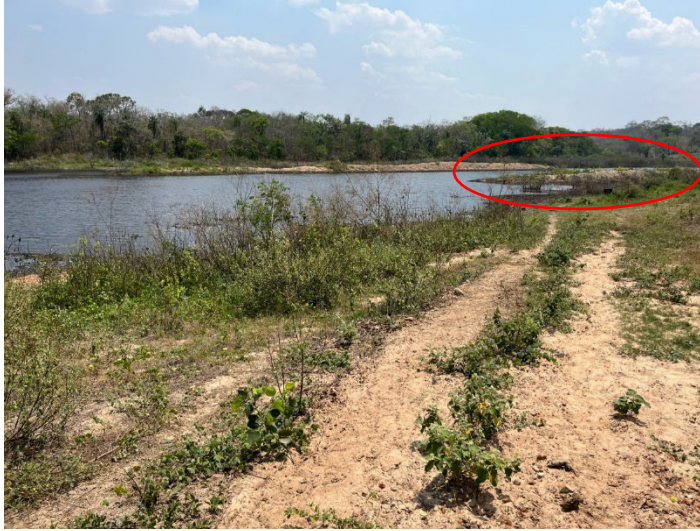
Picture 4: An atajado in San Fermín, San Rafael, where the community claims the Contractor left two large sediment dumps (one of which is circled).
