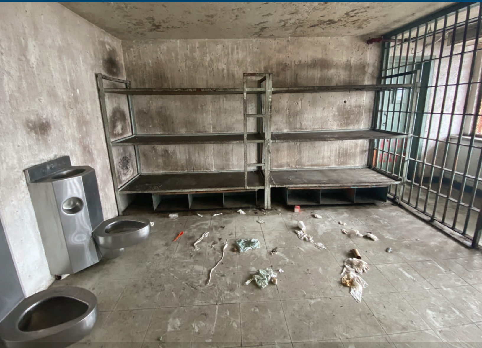
House of Detention, New Orleans (2020, closed 2012).
