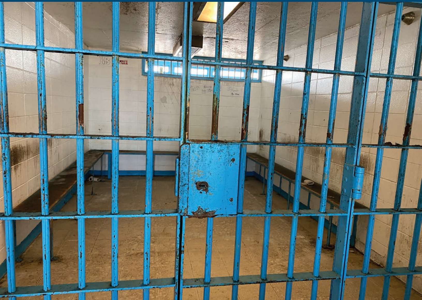
House of Detention, New Orleans (2020, closed 2012).
