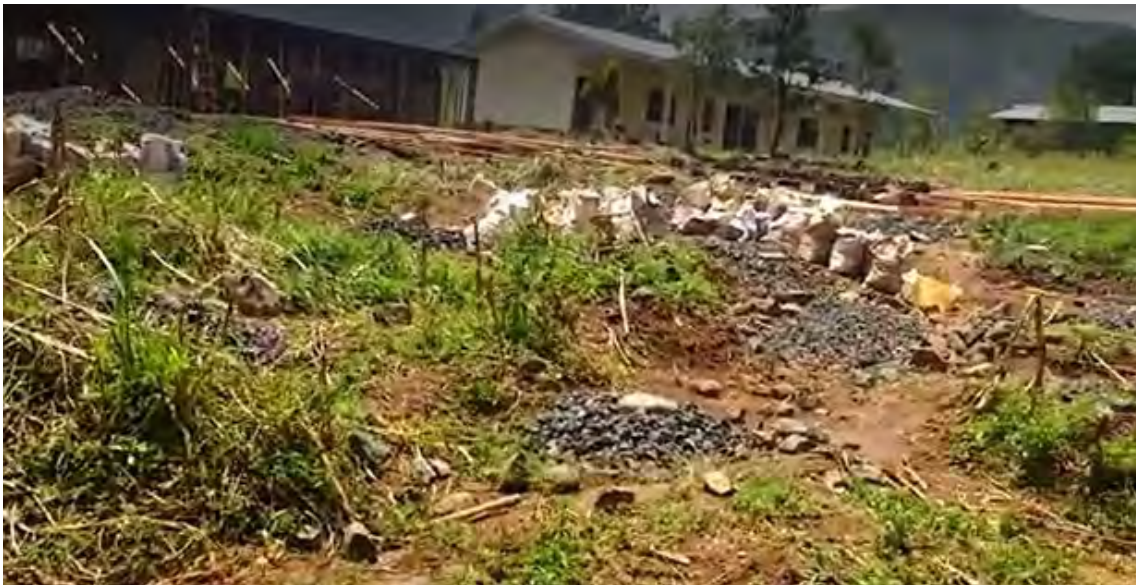
A view of the abandoned Government High School in Akeh village, a rural community in the North-West region. The school has been closed since July 2018. © Private, April 2021, Akeh, North-West region, Cameroon
