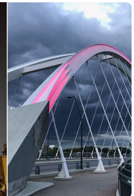
Lowry Avenue Bridge Minnesota, USA
