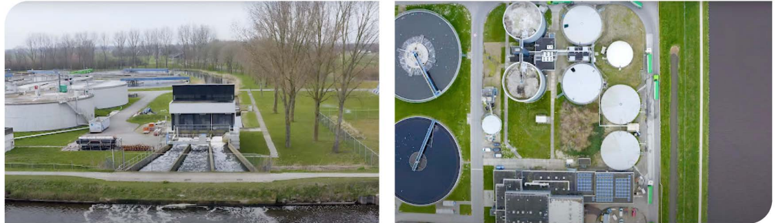
Caption: Intake structure from the Eems Canal (left) to the water treatment system (right) in Eemshaven, Netherlands, treating process water conveyed to Google’s data center.
