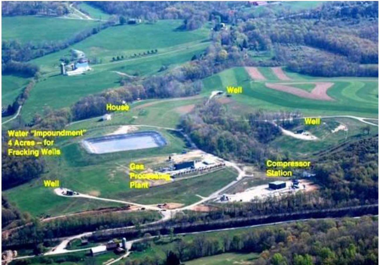
Figure B8.8 A shale gas production facility in the NE United States 14
