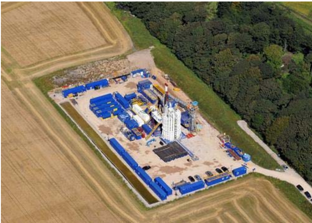
Figure B8.3 Hydraulic fracturing at Preese Hall, Lancashire UK 7
