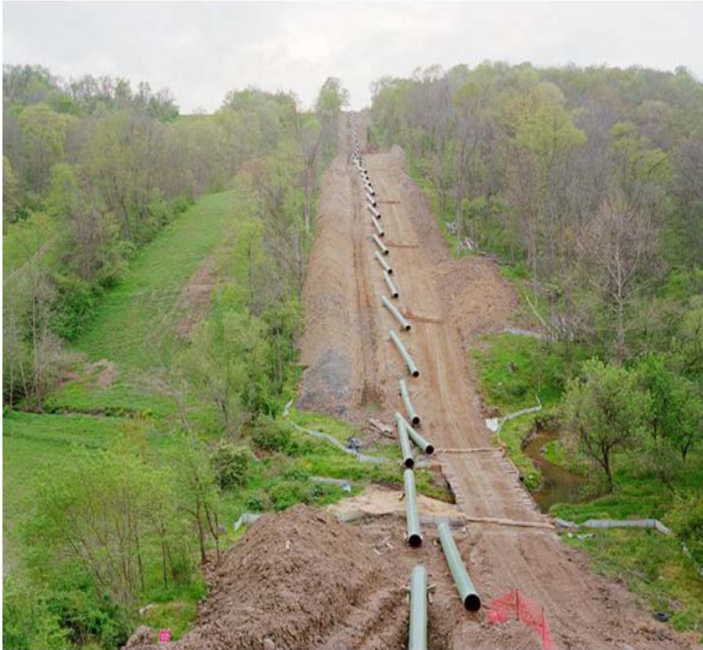
Figure B8.4 Pipeline construction in the NE United States 9
