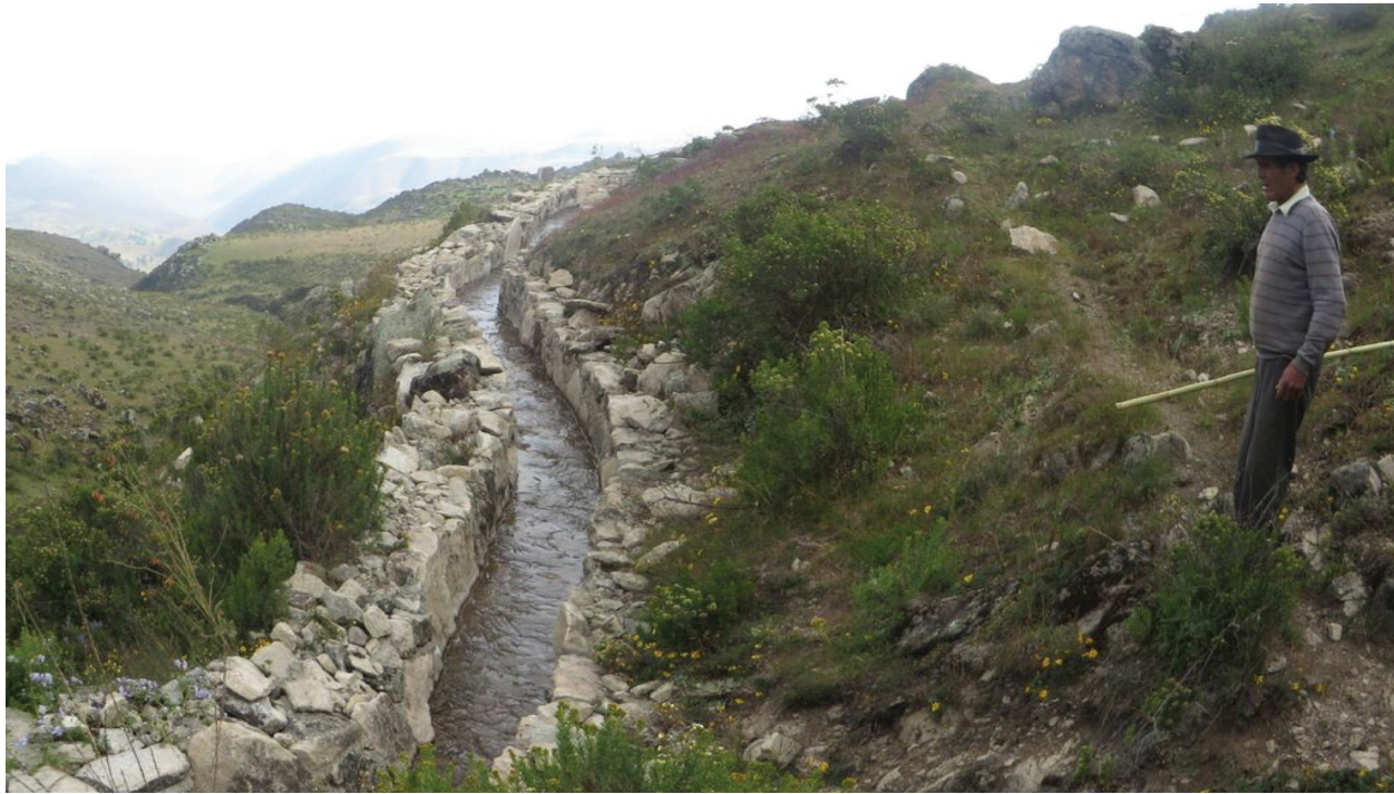
Photo 1: A restored mamanteo channel in the community, which is believed to “seed” water from the wet season for supply during the dry season. Photo: Leah Bremer
