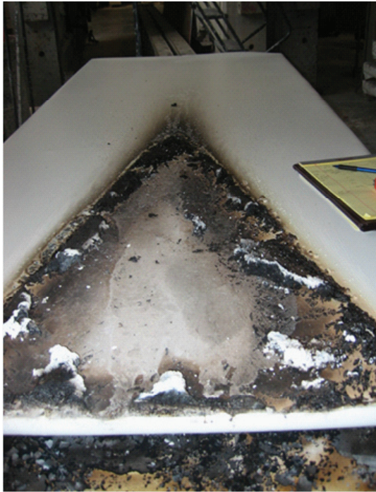
Photo 6 – PVC over Dens Deck
