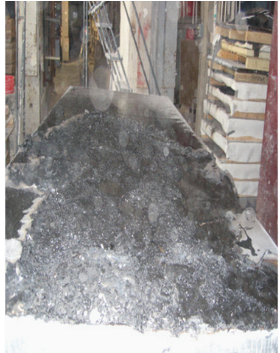
Photo 7 – FR rated EPDM over Iso, excessive lateral flame spread
