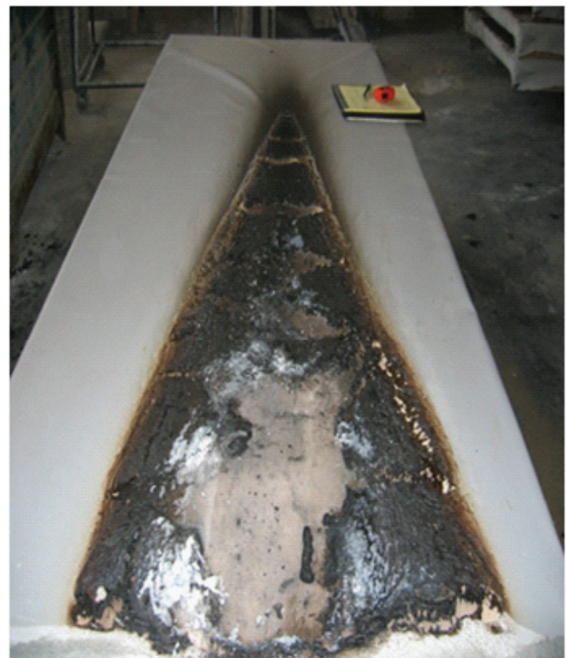
Photo 5 – TPO over Dens Deck
