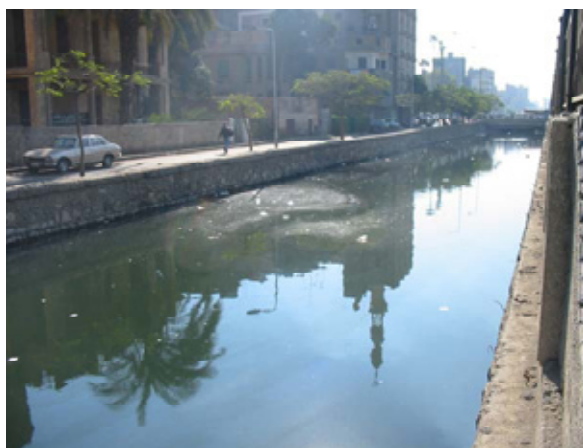
Photo 5.15: Water Pollution Status of Canal in Cairo
