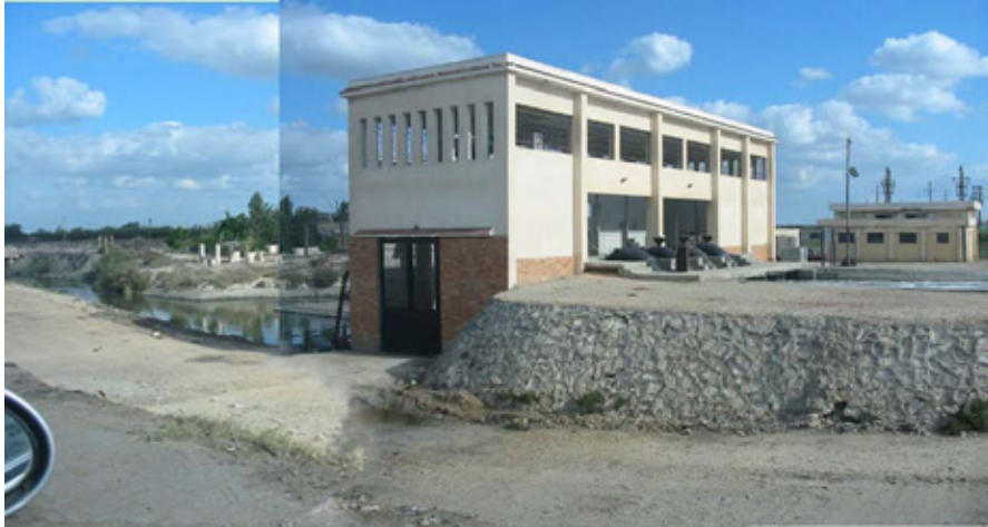
Photo 5.17: Pump Station at Alexandria
