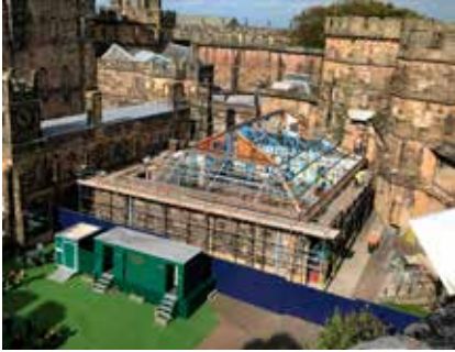
Conservation works, Lancaster Castle.
