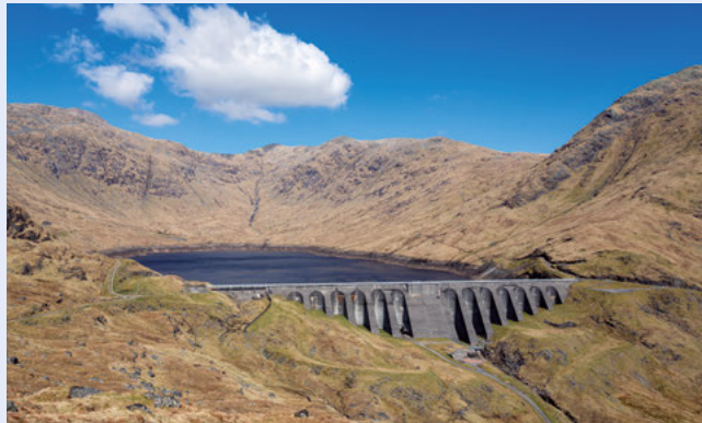
Cruachan 440MW capacity
