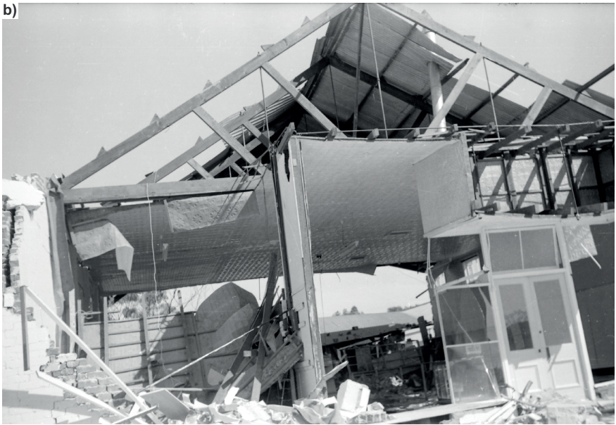
Figure 10. Examples of damage to infrastructure and the land: a) both the standard and narrow gauge rail lines were severely warped; b) houses and public buildings were extensively damaged or destroyed, although the framework of some houses remained upright; c) fences were offset across the fault; d) farmers had to deal with sizable fractures that opened in their paddocks (see next page)
