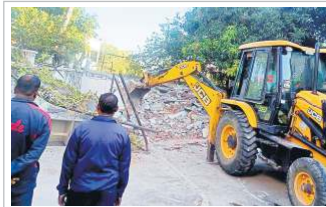
Bulldozer razing a 4-km compound wall in Pocharam municipality on Saturday
