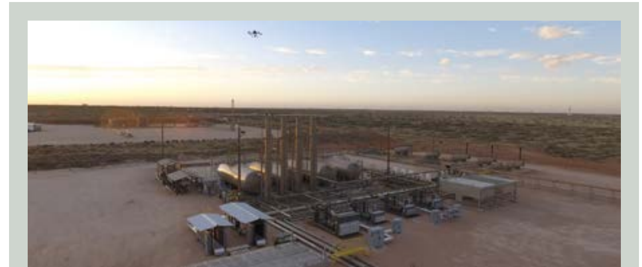
Drone performing voluntary OGI inspection on a Coterra tankless facility in the Permian Basin
