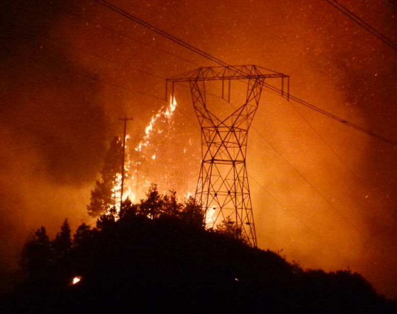
Fire threatening power lines running along US 97 in Washington State. WA State Department of Transportation
