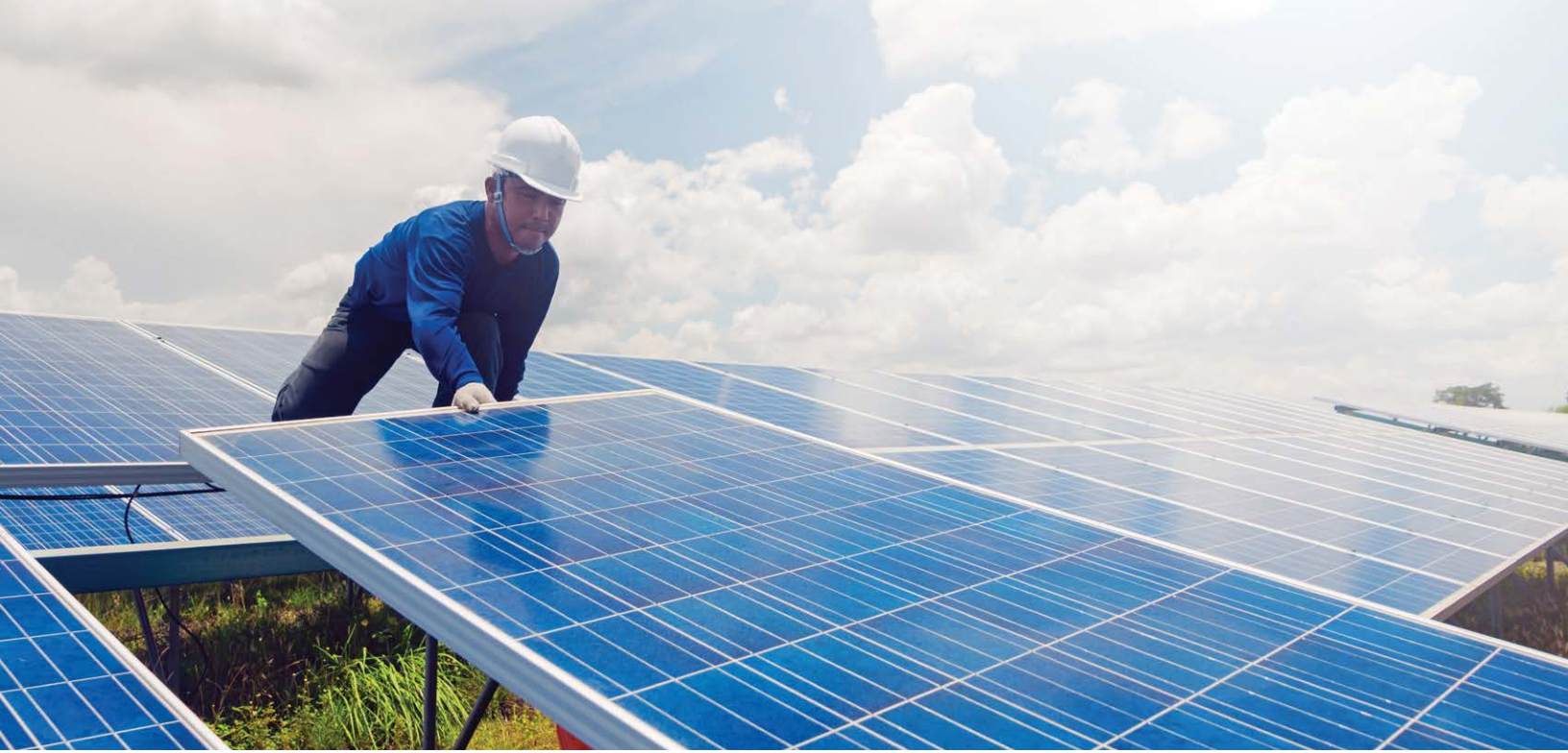
Engineer installing solar panel.
