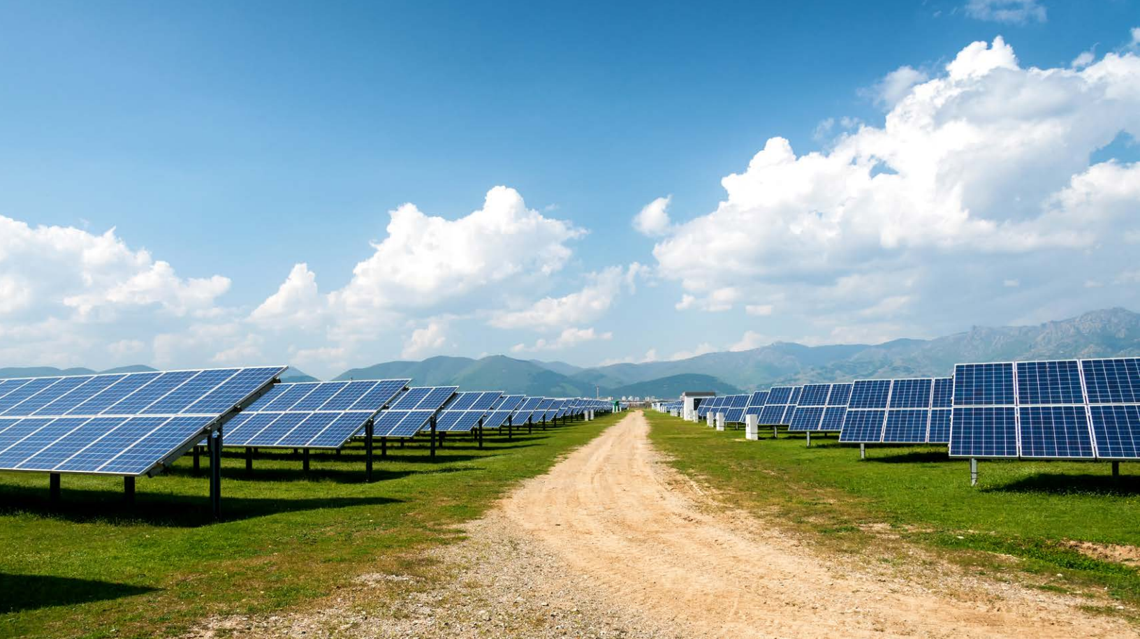
Panoramic view of solar panels.
