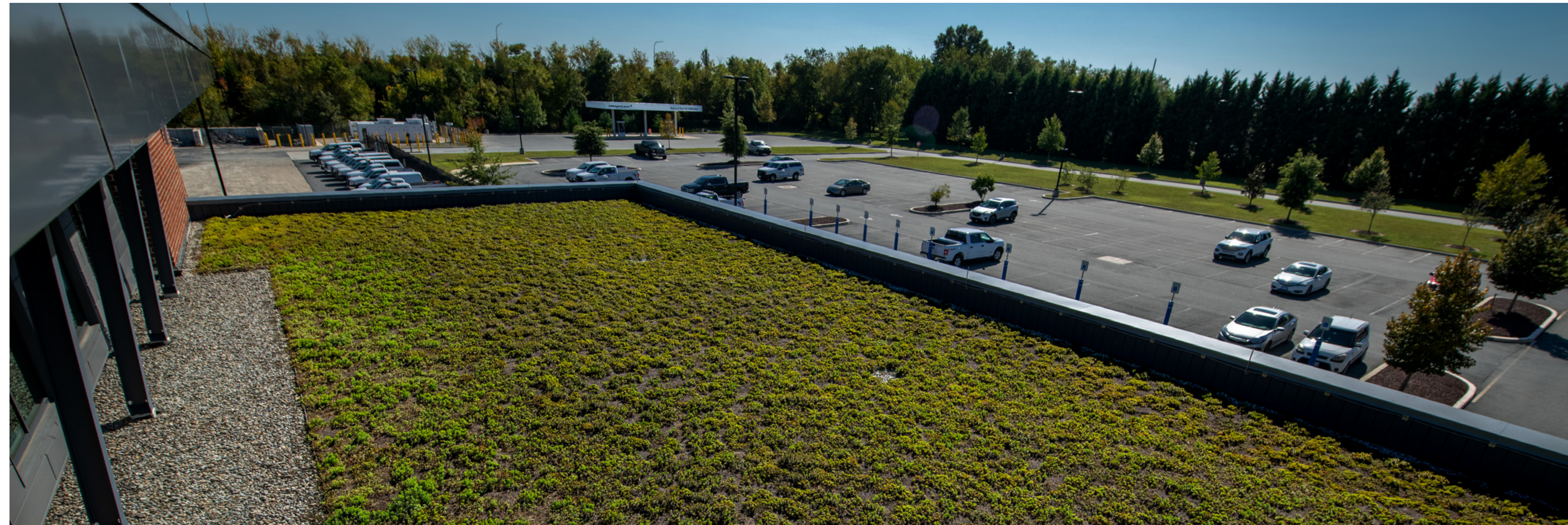
Our Energy Lane office building, home to our corporate headquarters in Dover, Delaware, has a living roof and walking paths on site. The Green Building Initiative awarded the building the Green Globes Certification, a national recognition for capturing a higher standard of environmental integrity.
