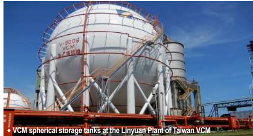
• VCM spherical storage tanks at the Linyuan Plant of Taiwan VCM
