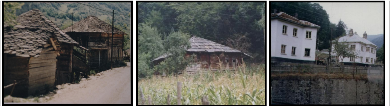
Photo 14. Traditional stone and shingle covered wooden buildings and management buildings constructed by Belgians at Zindan valley in area of Ayancık.
