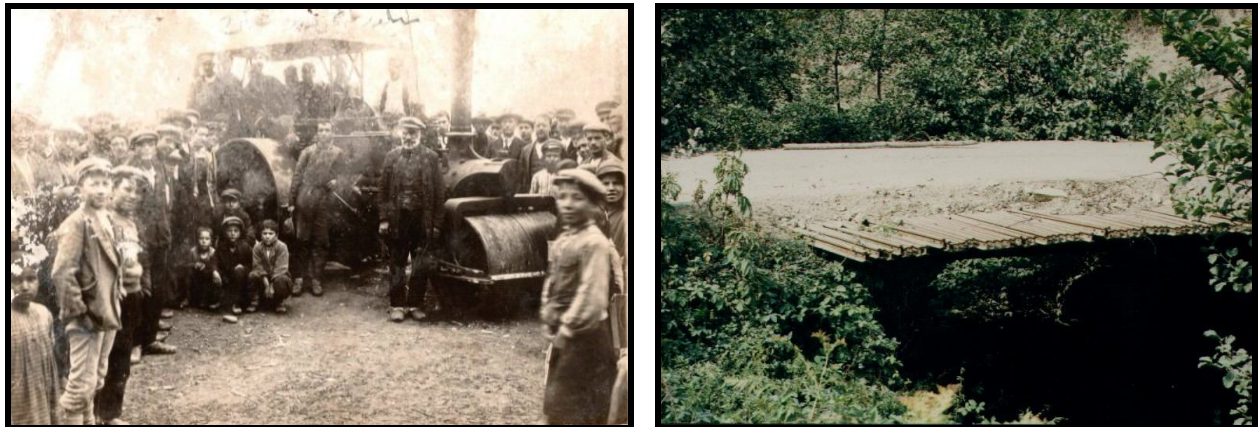
Photo 9. After the flood, a network of roads was installed in the forests (left) (ANONYMOUS) and the old rails were used for constructing the bridges (right).
