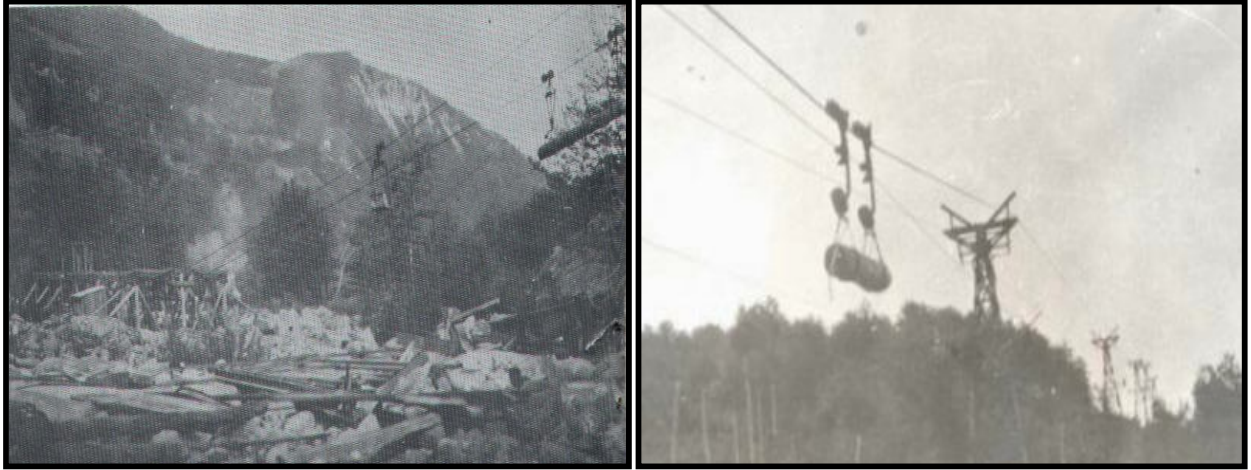
Photo 2. Lumber transportation via teleferic line from Çangal Mountains to Ayancık Lumber Factory in 1930's (ANONYMOUS).
