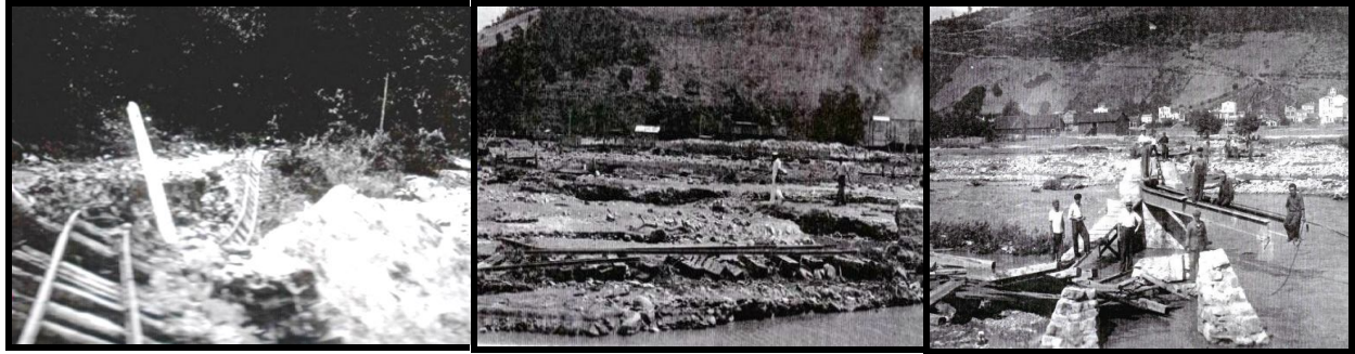
Photo 8. The flood that occurred in 1963 destroyed the all transportation system from the Zindan and Çangal forests to the district center of Ayancık (ANONYMOUS).
