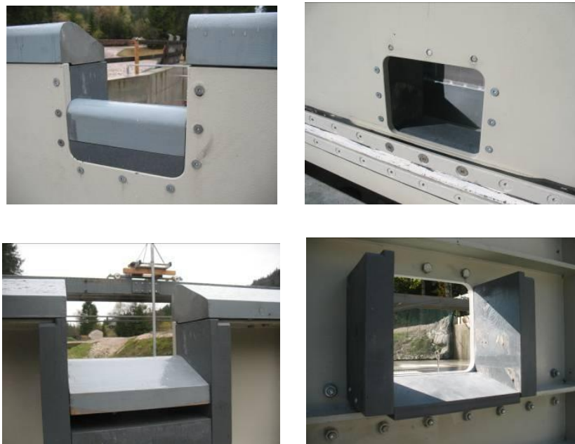
Figure 4: Fish downstream migration opening variants: Surface near (left column) and bottom near (right column) positioning seen from the head water (top row) and from the tail water (bottom row)
