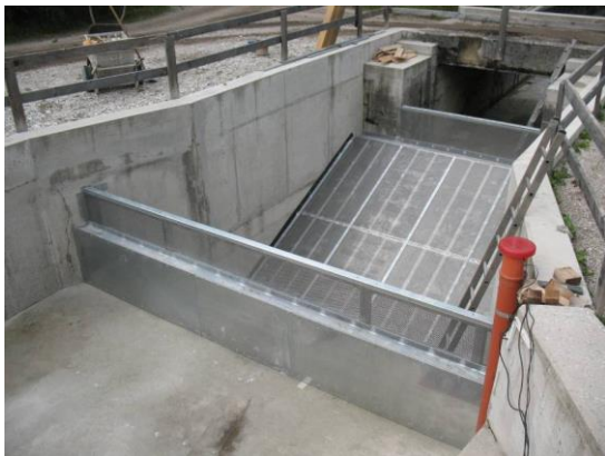
Figure 5: Fish barriers in the test setup: Schematic diagram (top – fish barriers represented as red lines), net installation upstream the test section in 2013 (middle – left) and the corresponding fish barrier in 2014 (middle – right), arrangement of metal plates in the tail water area (bottom – left) and the fish retrieval flume at its downstream end (bottom – right); Flow direction from the left to the right
