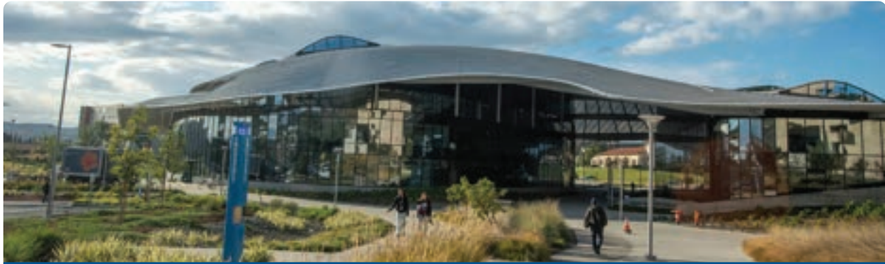
CPP Student Services Building
