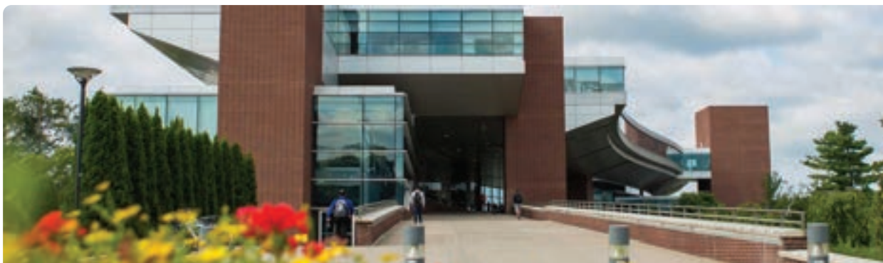
Westgate Building, Penn State University Park
