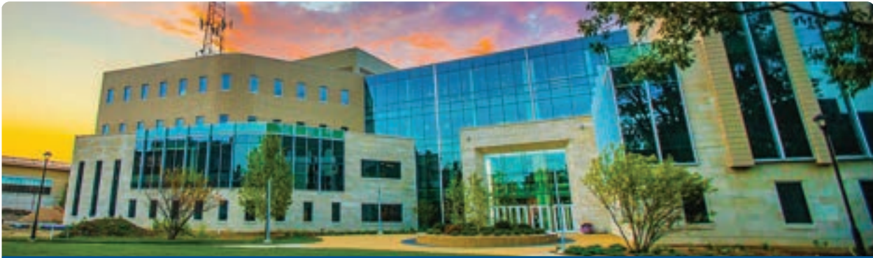
Business and Engineering Convergence Center
