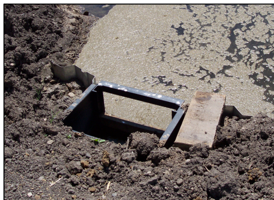
Newly constructed stop-log structure
