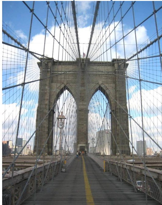
The Brooklyn Bridge provides access between Manhattan and Brooklyn.
