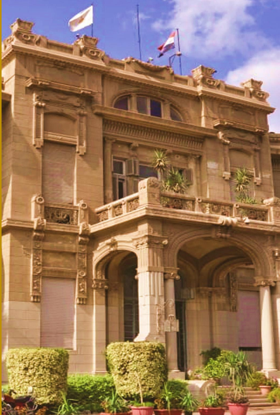
Al-Zaafaran Palace Entrance
