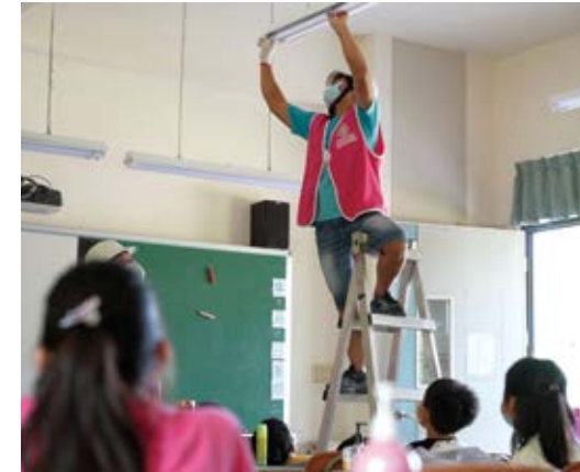
Campus LED installation projects
