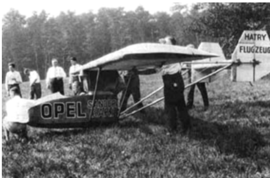
It was in the Rak 1 airplane that von Opel finally made a rocket-powered flight, achieving around 90 mph on Sept. 30, 1929. The aircraft didn't survive the landing, but von Opel did. Apparently satisfied, he walked away from rocketry.
