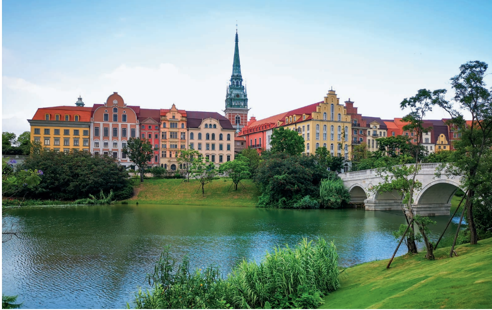
The Huawei Employee Training Center at Sanyapo
