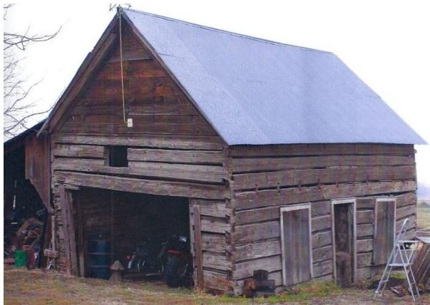
The Prince's Cabin, 2008, before moving and restoration at Frenchtown
