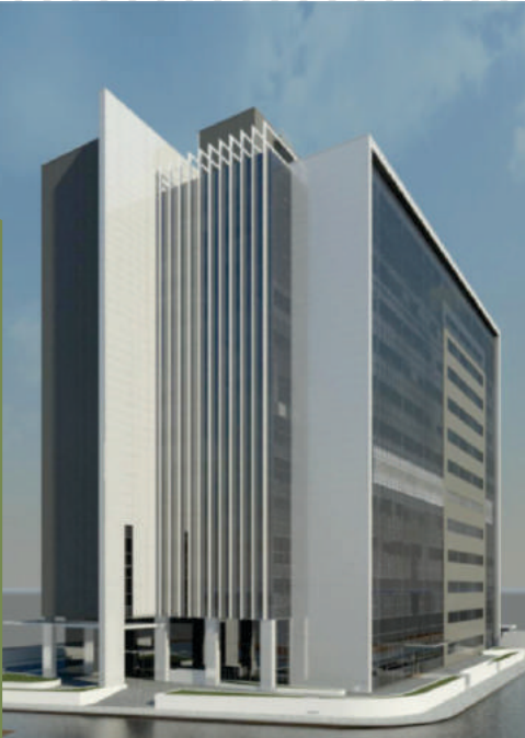
Hospital São Luiz, São Caetano, SP Under construction
